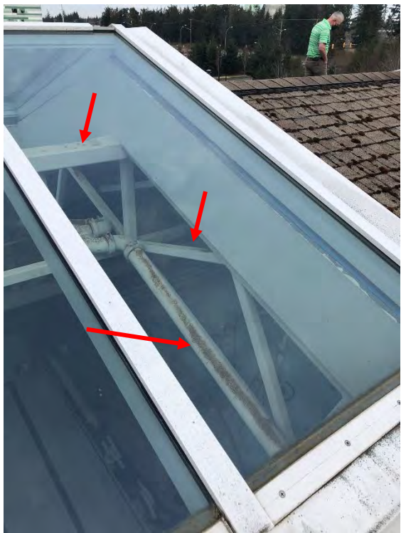
Photo 13 Roof truss and roof drain lines
