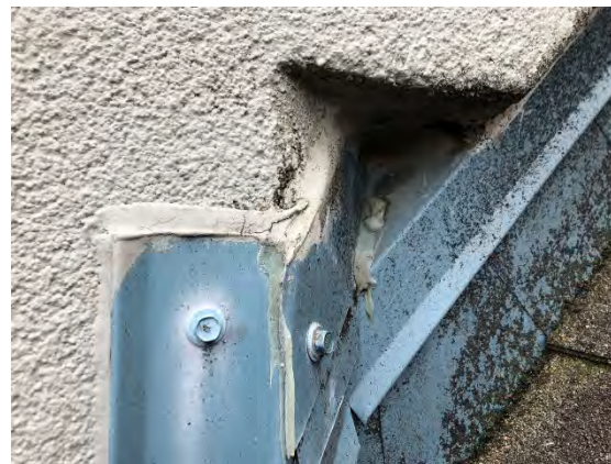
Photo 19 Typical roof saddle detail
