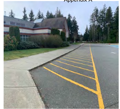
Photo A1 Paving and curbing in good condition.
