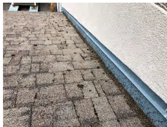
Photo 12 Staining on roof truss
