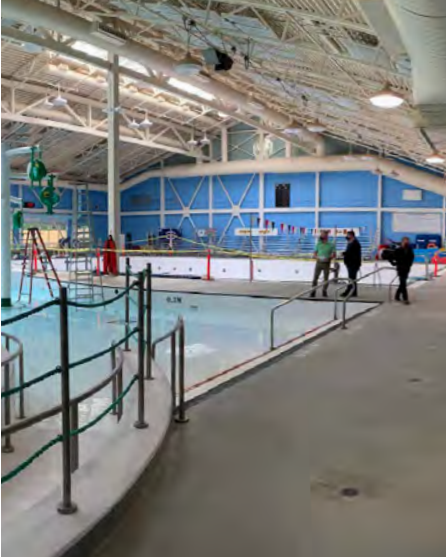
On site review March 17, 2021
