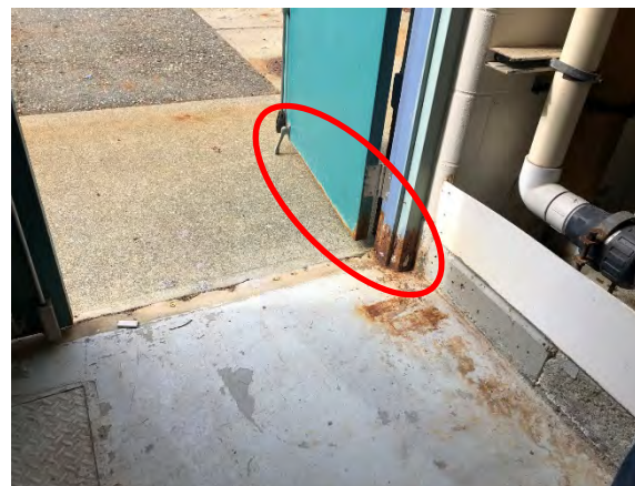
Photo 6 Mechanical room, south elevation
