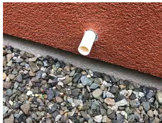
Photo 4 New pipe penetration at electrical room, west elevation
