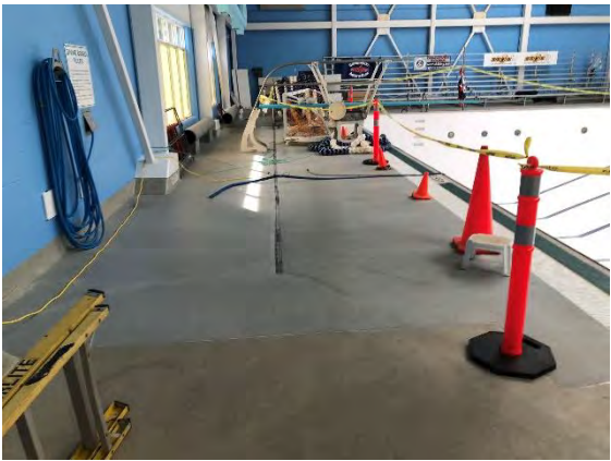
Photo 6 Area of renewed coating at pool deck
