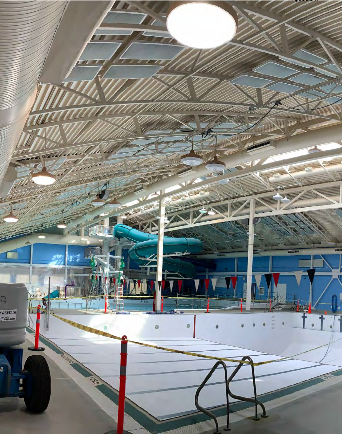
Image 1. Natatorium during Consultant Facility Review March 17, 2021
