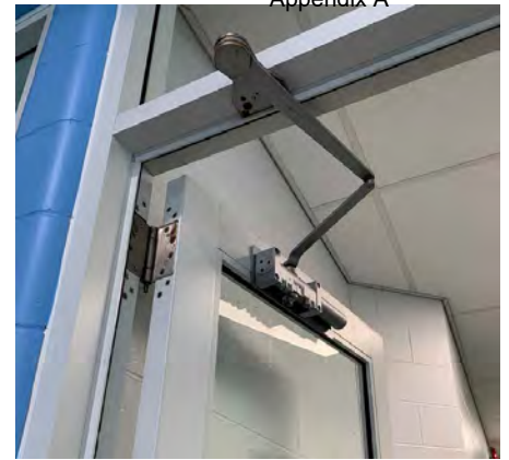
Photo A7 Interior doors at natatorium
