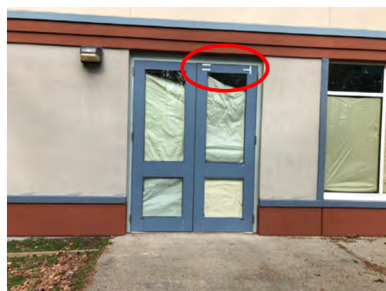
Photo 5 South elevation natatorium exit door
